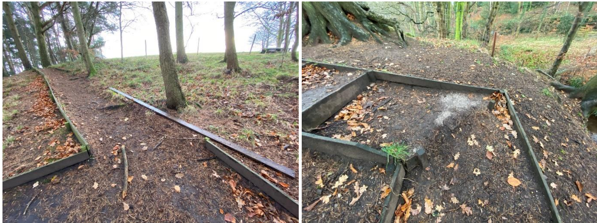
Figure Four: Sections of the path in the upper section of the woodland where boards require replacement
